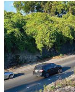
Overgrown vegetation hanging < 16.5 feet over paved shoulder
