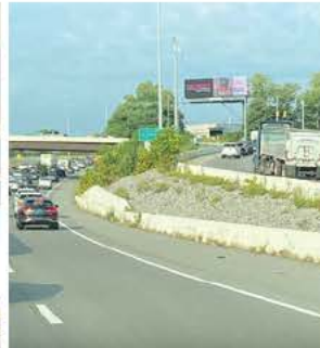
Overgrown vegetation along rip-rap slope
